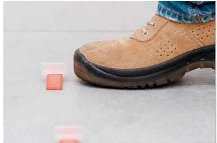
Once the adhesive cement has set, to remove the clip you simply need to tap it with the rubber mallet or the tip of your toe in the direction of the joint.
