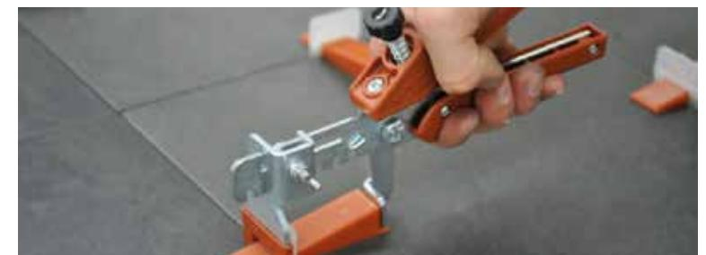
2. We recommend the use of adjustable traction pliers to make this task easier.
